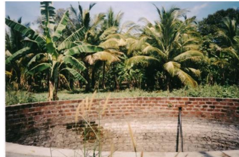
Figure 2: A Lined Agro-well in the Belikulama tank cascade
